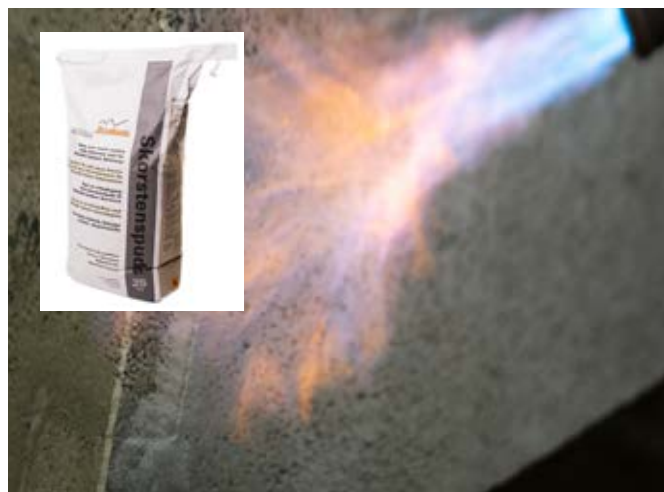
Burn off the fibres on external surface before rendering.
